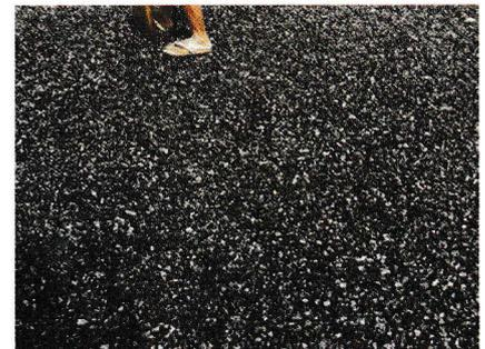
On 27th January, 2010 Cochin Corporation under the supervision of BPCL has constructed a stretch of asphalt road using plastics waste at Kaloor Manapatty Road. The plastics waste was shredded by CREDAI Clean Kochi Movement for Road Tarring.
