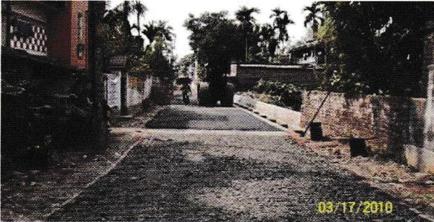
Road laying using plastics waste under progress
