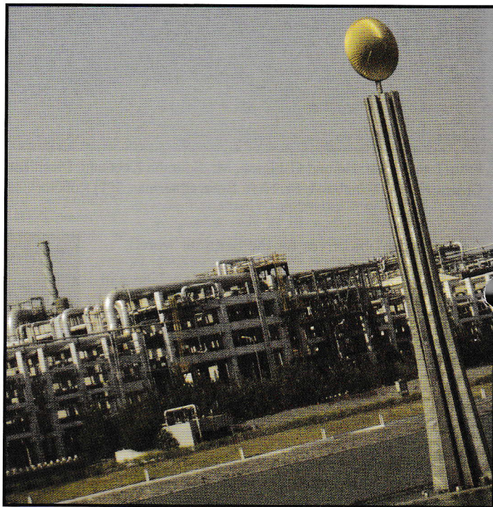
A View of the Plant of Reliance Industries Ltd., Jamnagar, Gujarat
