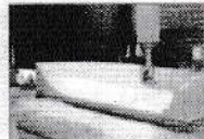
Engineered putty applied over the foam is machined to finish the direct to mould hull.
