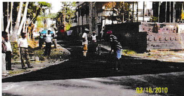
Seal coat being laid
