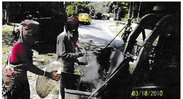
Plastics waste being spread over aggregates
