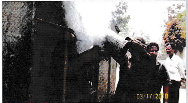
Hot bitumen being added to the heated aggregate – plastics waste mix
