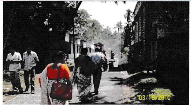
Selected road for laying
