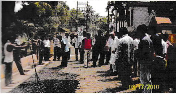
Road under construction
