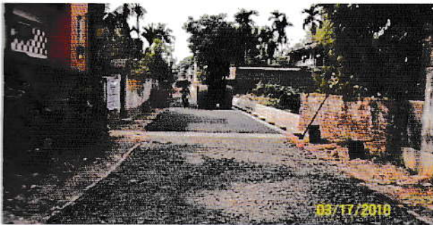
Road laying using plastics waste under progress
